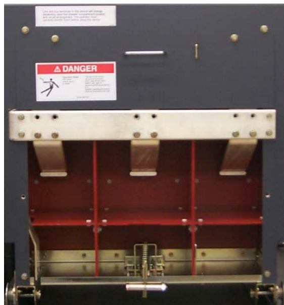
Figure 2: Device shown with lower terminals grounded Torque .375-16 (Grade 5) Hardware to 20ft./lbs.
